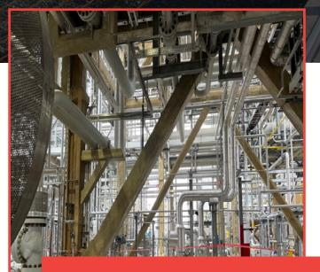
Geopolymer Solutions' FP250 supports major Texas Gulf Coast oil company with passive fireproofing for structural steel beams, vessel skirts and equipment supports.
